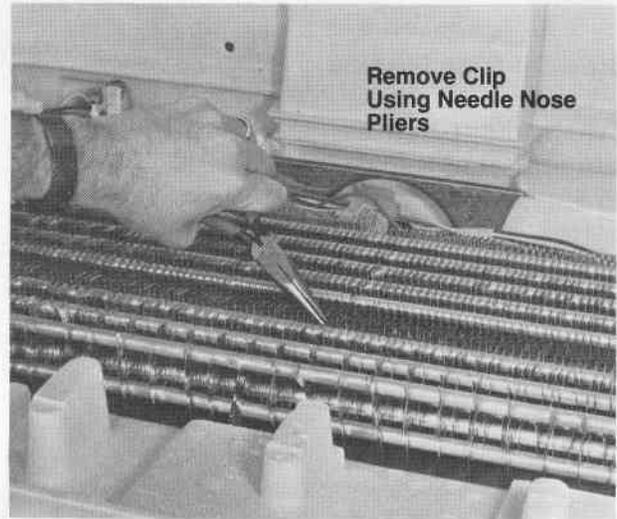
8. Pull the shield and the heater out.
