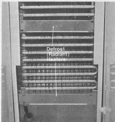
The defrost timer energizes the defrost heater every eight hours of accumulated compressor run time. When the temperature in the thermostat area reaches approximately  $+40^{\circ}$  F the thermostat contacts open the circuit to the defrost heater.
