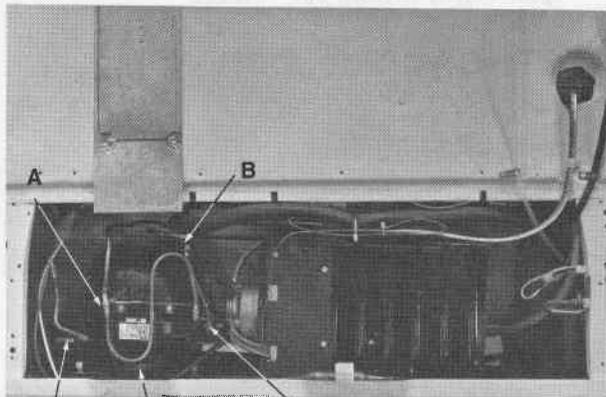
Process Tube    Discharge Tube    Suction Tube    Side-By-Side
