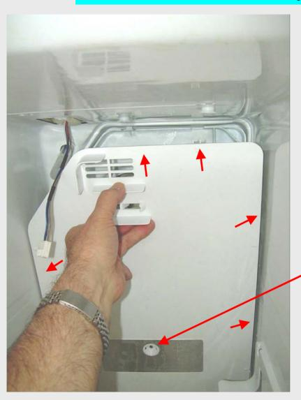
To access evaporator, remove the evaporator back panel.
