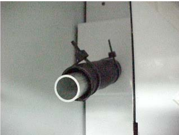
Figure 2 – Sleeve must cover entire heater section outside metal cover. Trim sleeve length, if needed.
