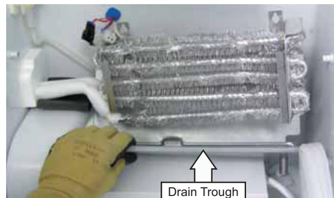
**Note:** When installing the drain trough, insure trough outlet is inserted into the drain funnel.
