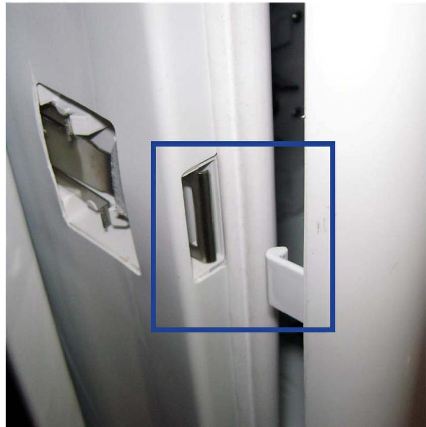
**Simple design as metal “catch” bends in and out to secure and release door strike**
