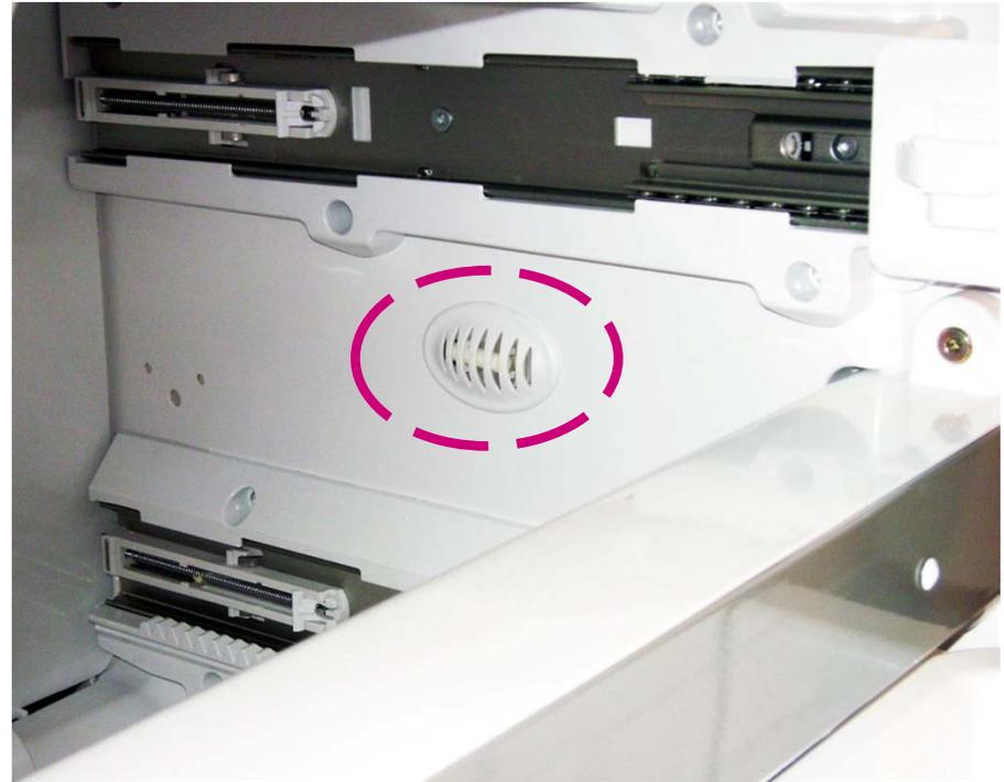
FZR Thermistor located on right side wall
