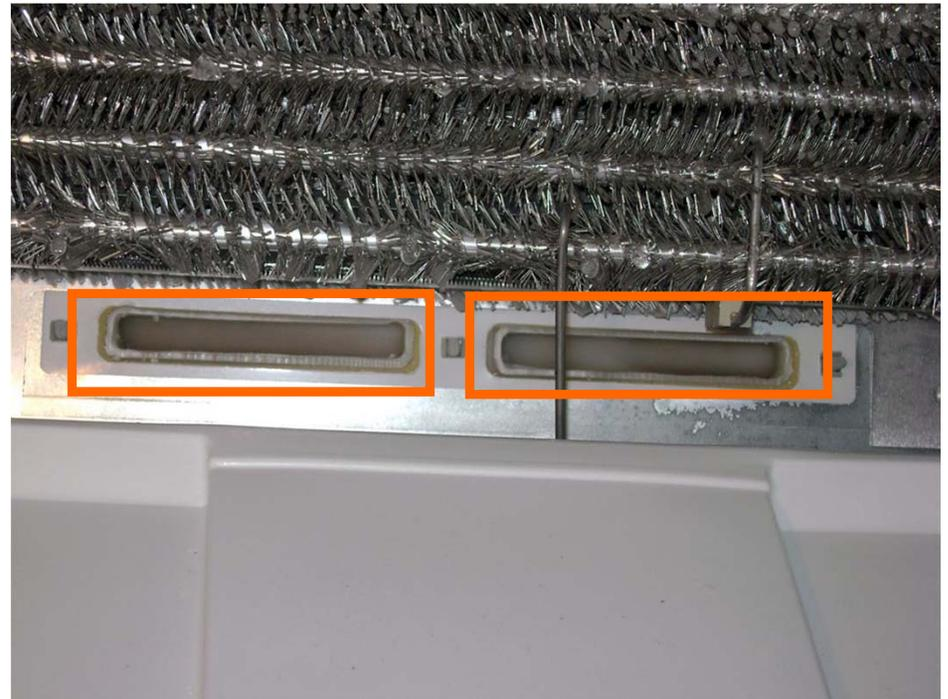
440  $\Omega$  Return duct heaters. Not replaceable
