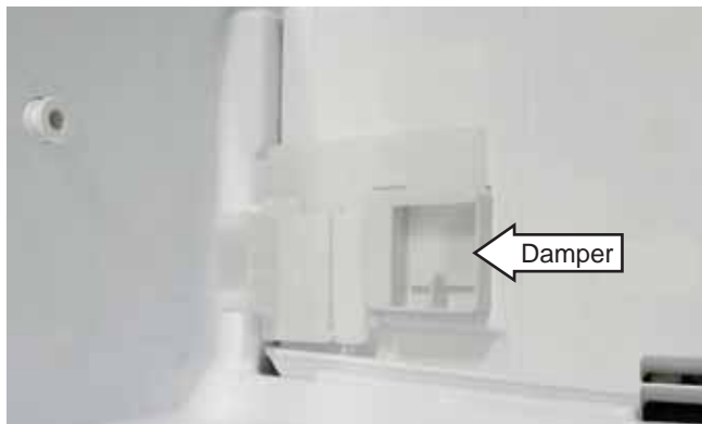
Damper shown in closed position
