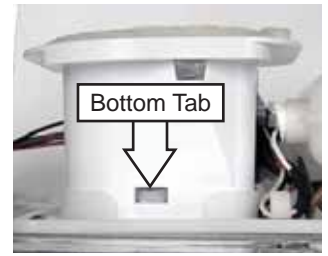
Bottom View of Duct
