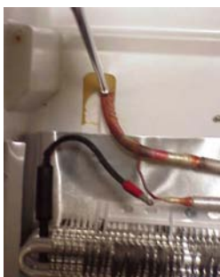
Cut suction line off at liner. Remove evaporator and save for reuse.
