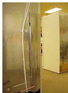
Using screws in kit, attach cover to back of cabinet. Line lower cover up with top of machine compartment opening
