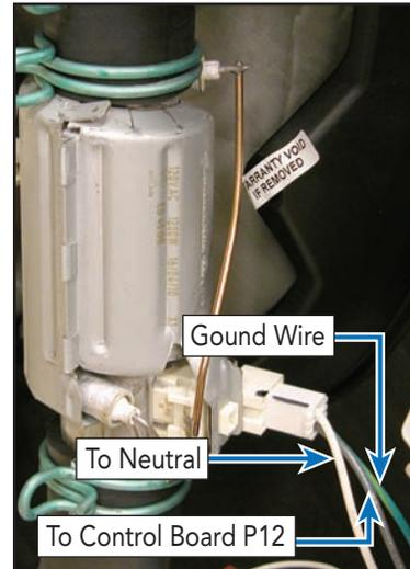
connector that supplies power to the heating element and the ground wire which connects to a spade terminal on the heater housing. Image to left shows the connections.
