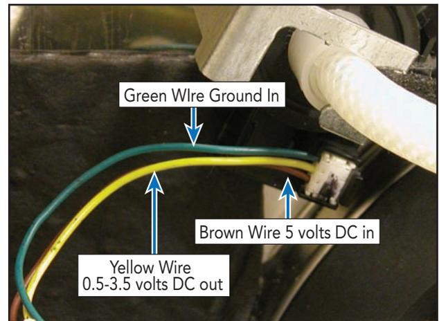
As the water level increases, the pressure in the 1/4" (.63 cm) pressure tube, connected to the level sensor input, increases as well. This pressure causes an internal amplifier to vary the output voltage to the board. An empty sump should produce a reading of .5 - .8 VDC between J9 – 4 and ground while a full sump should read approximately 3.5 VDC. Depending on the water level, the output voltage to the control board changes and is processed in the board.
