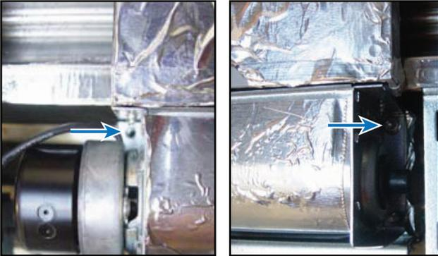
To access the remaining two screws, the right side air/water Inlet assembly will need to be removed.
