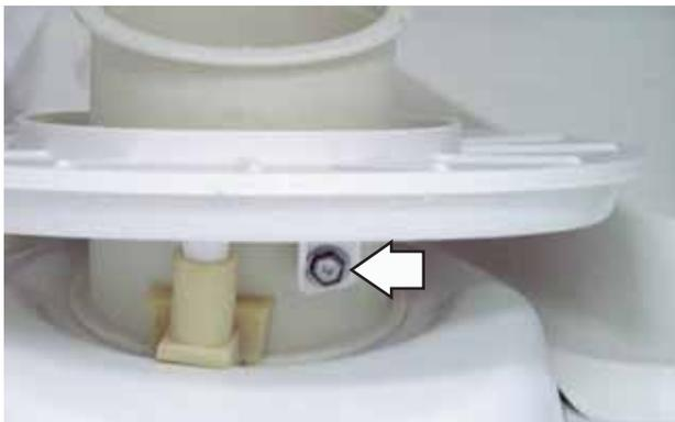
4. Gently push the same tab in to lift the fine filter assembly up and out. (See step 2.)
