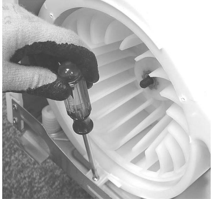
10. Remove the blower attachment screw under the Thermistor.
