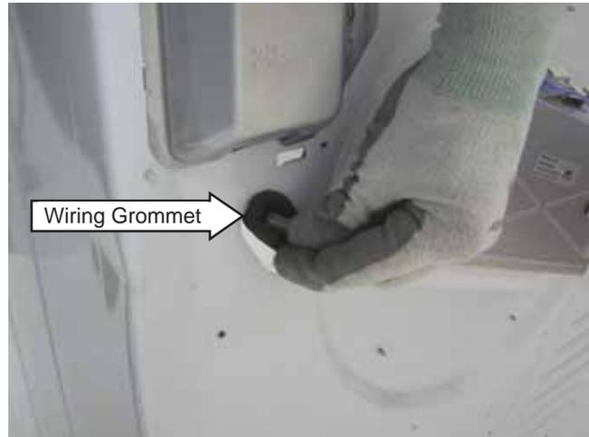
6. Pull the wiring thru the wiring entry opening.
