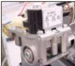
Split-coil gas valves have a regulator, 3 coils (holding, booster & secondary) & 2 valves (dual & secondary).
