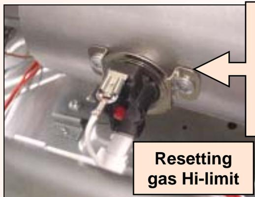
**NOTE:** Hi-limits (high temp cutouts), located on heater/burner housings, trip @ **347°F (electric)** or **347°F (gas)**. To reset Hi-limits, press **red** button.
