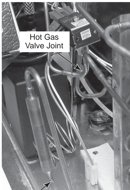
Drier Filter Capillary Tube
