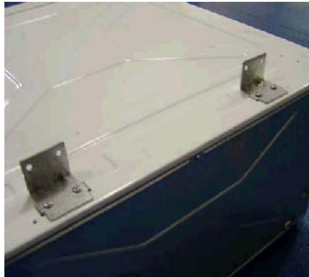
3. Remove the front service panel from the washer. Using two or more people, carefully lift the washer onto the pedestal and set flush against the rear brackets as shown.
