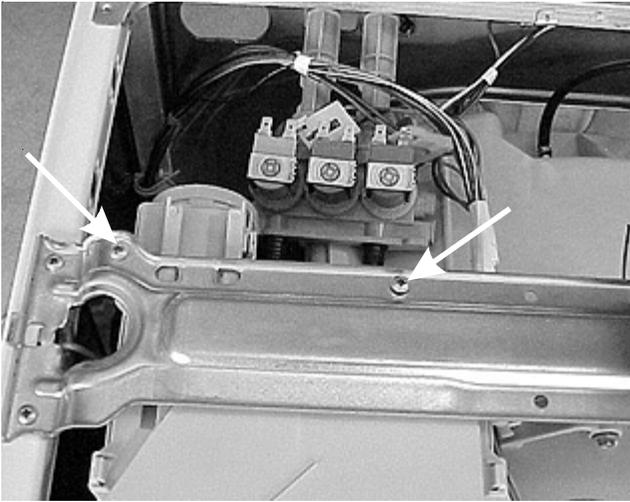
8. Slide the housing back until the tabs of the center cross bar release and the housing drops down.
