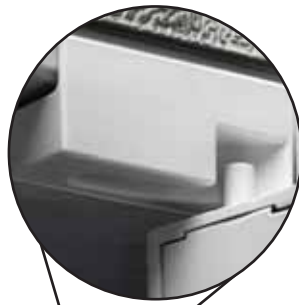
Door Opening - Pin Exiting Track
