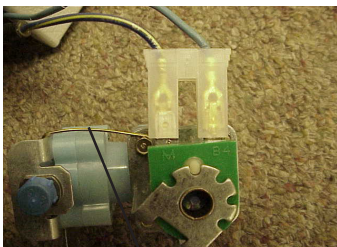
Terminal on Coil is Installed
