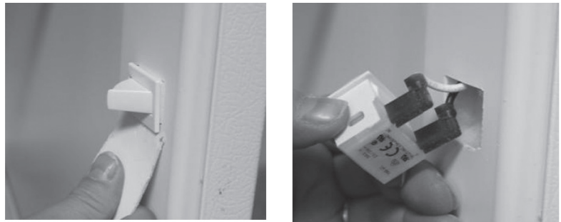
Cabinet wall location
