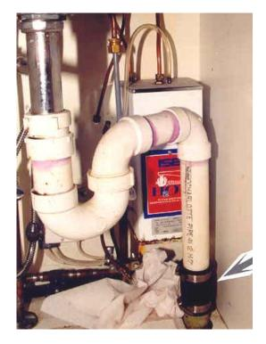
If the piping is old heavy galvanized or the drain disappears into the wall and cannot be lowered, you are in for trouble. Galvanized piping requires cutting and threading unless a rubber coupling is used. Cutting galvanized piping is always difficult. The simplest solution may be to fit in one of the smaller Badger models or a brand with dimensions similar to the original.
